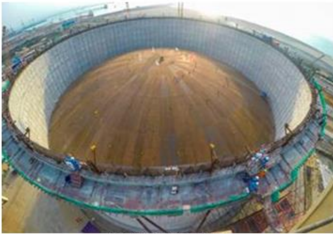
Roof raising in progress.
